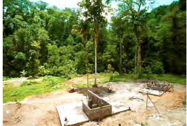
Construction site, April 1994
