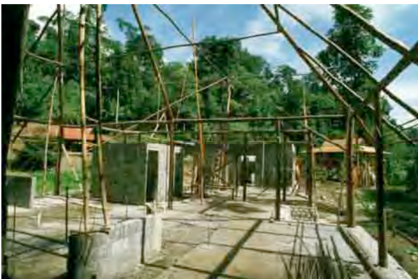
Construction site, July 1994
