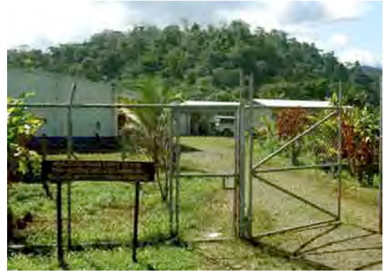
The primary school in the center of La Gamba houses three classrooms for 80 students.
