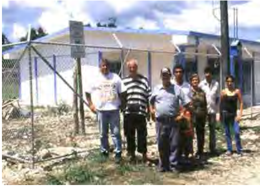
The Health Committee of ASOPROBI with Michael Schnitzler and Ana Catalina Torres in front of the Puesto de Salud. The building has a waiting room, a surgery room, a doctor's room, a toilet and shower.
