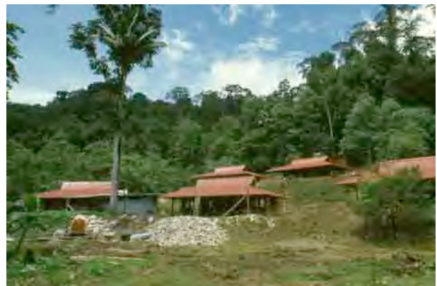
Construction site, November 1994
